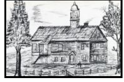
To the East you would have seen a "Gemeinhaus"... a building for worship and lodging for students and village visitors....
