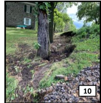
**Photos 8-10...**Raging water tore away the fence line in front of the house and eroded a very large area at the bank along the tracks with water level shown by debris at tree.
